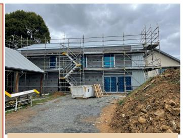
Three sides of the homestay and roof have been clad in corrugated iron. The front will feature vertically mounted timbers milled from the demolished Charleyong bridge.
